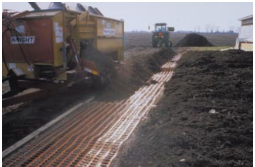
Biofilter under construction: placing biofilter material on top of the ducting.
