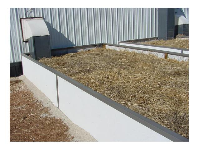
Figure 1. Biofilter at OSU Swine Research and Education Center filled with wheat straw. Notice grouting at bottom to keep airtight.
